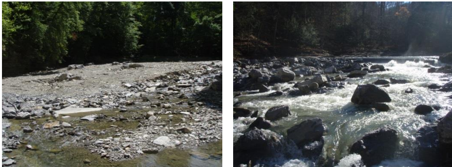
Figure 2c-2. Rock ramp on the uppermost dam post-construction and pre-flood, and after the Superstorm Sandy flood.
