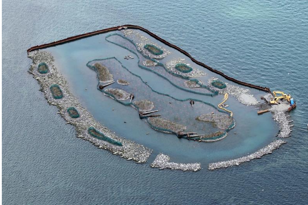
Figure 2c-1. Aerial View of Frog Island near completion. Photo: Paul Leuchner
